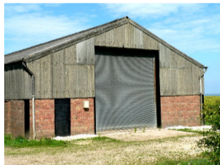
Moiré on the garage door
